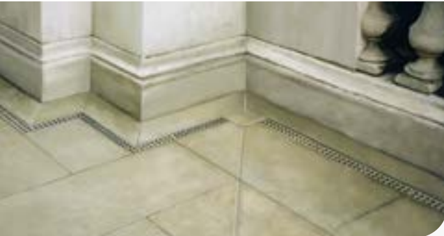
Custom made gratings Cast iron grating and show edge coupled with stainless steel channel provided a complete drainage solution to blend with the period architecture at Somerset House, City of Westminster.
